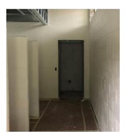
Figure 3 Carver – Block fill and first coat
